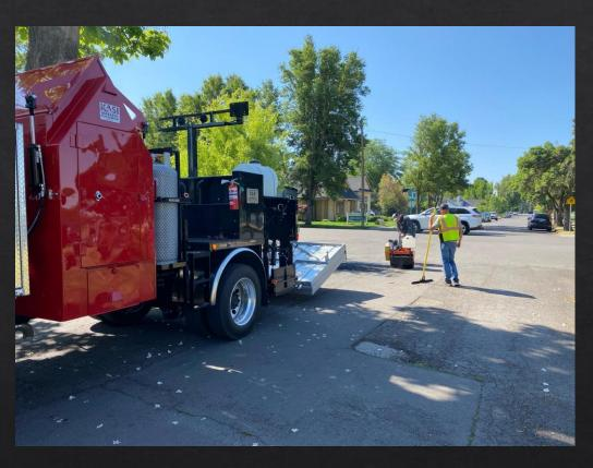
Light the Infrared Chamber and position the heater over the repair area
