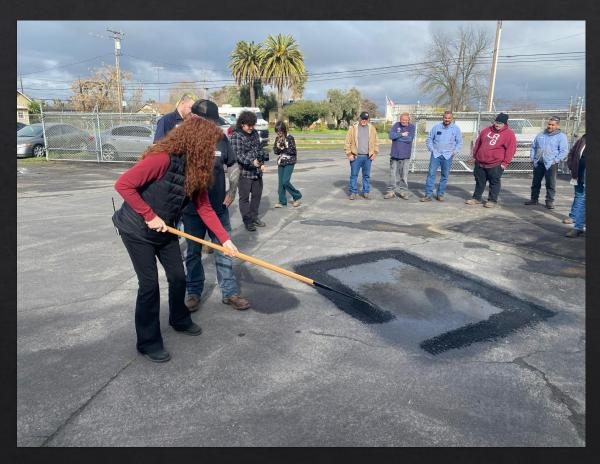
Once the existing asphalt has been adequately heated, begin to scarify the repair area.
