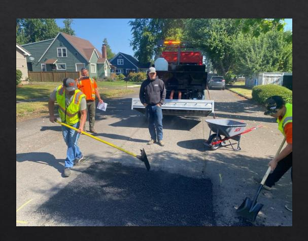
Once you have finished scarifying and adding rejuvenator – it is time to add new asphalt from the hotbox on the truck. The amount of new asphalt that you add will be dependent on the type of repair you are completing. Bigger holes require more asphalt. Make sure to lute the fresh mix out smoothly and leave a  $\frac{1}{4}$ " –  $\frac{1}{2}$ " above grade around the edges for compaction.
