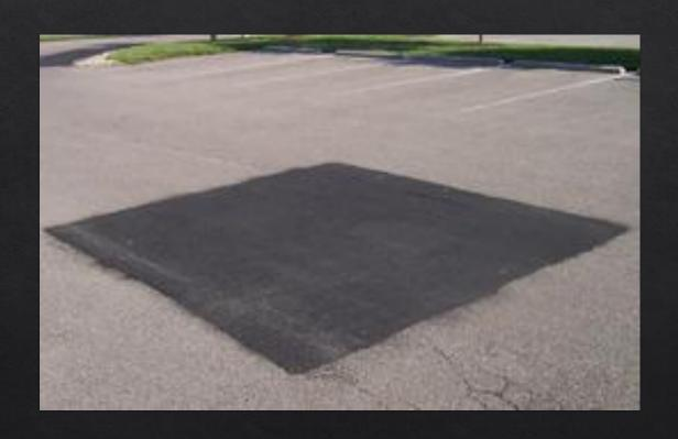
The finished product should look very similar to a saw cut and replace patch. Attention to your edge details, proper luting, and proper compaction are all key elements that effect the aesthetics and look of the final patch.
